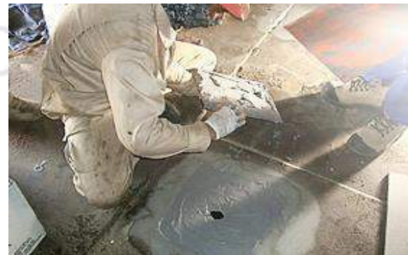
Repairing internal bottom of flow wash tank in Rumaila/BP
